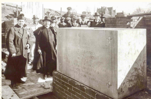
14 February 1923, the Foundation Stone
