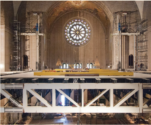
Steel deck of the scaffolding hoisted by workers
